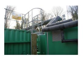
NAPL is recovered from abstraction wells using a technique of groundwater pumping to lower the head in the aquifer together with total fluids pumping using top filling pneumatic pumps. A relatively low vacuum to the well head enhanced NAPL recovery during the pilot test and was incorporated in the full scale design.
