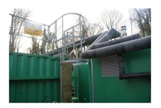
NAPL was recovered from abstraction wells using a technique of groundwater pumping to lower the head in the aquifer together with total fluids pumping using top filling pneumatic pumps. A relatively low vacuum to the well head enhanced NAPL recovery during the pilot test and was incorporated in the full-scale design.
